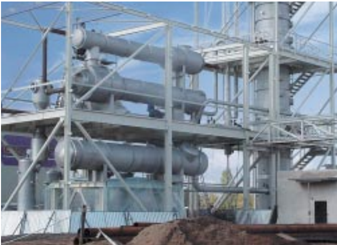
A single-effect ethanol distillation plant, shown during construction
