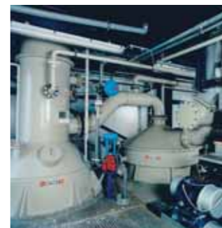
Vacuum cooling crystallizer for copperas
